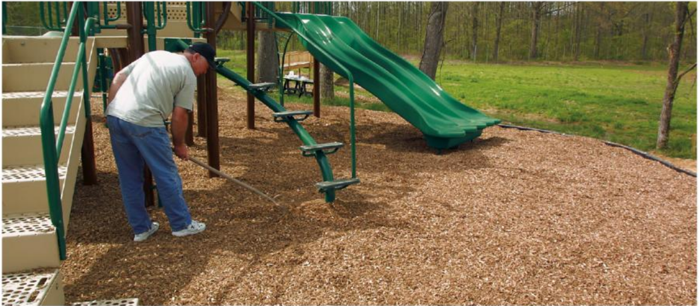
Raking loose-fill engineered wood fiber material
