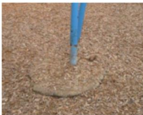
Exposed concrete footing (others)
