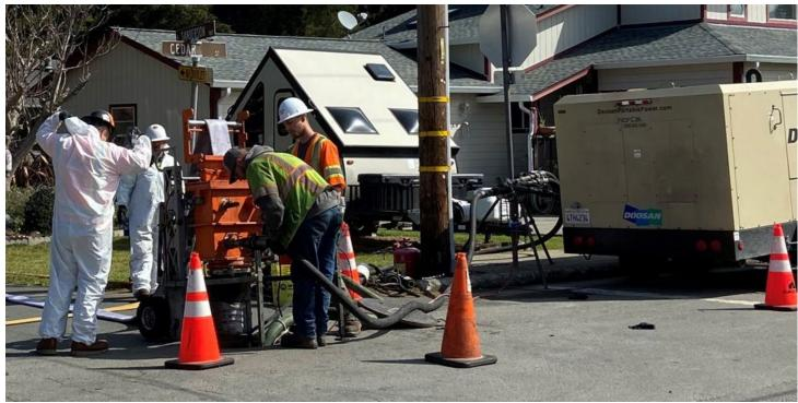
Another project that the City embarked on was the 2021 Cure-in-Place Pipeline. This important project rehabilitated approximately 9,480 linear feet (1.8 miles) of existing sewer pipe by lining internally via a cure-in-place process throughout various locations within the City. This project was funded by internal funds and a cost of \$192,000.
