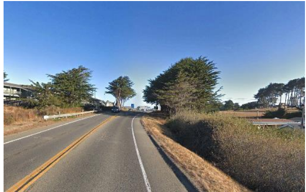
Figure 28: Narrow shoulder on Highway 1 between Airport Road and Pudding Creek Road (Source: Google Street View)
