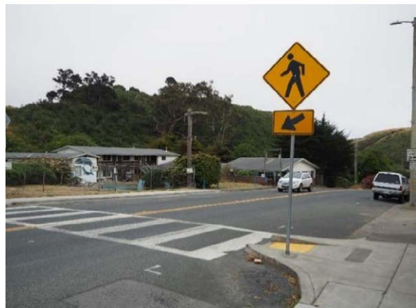
Figure 6: Existing Main Street crossing near Mill Street
