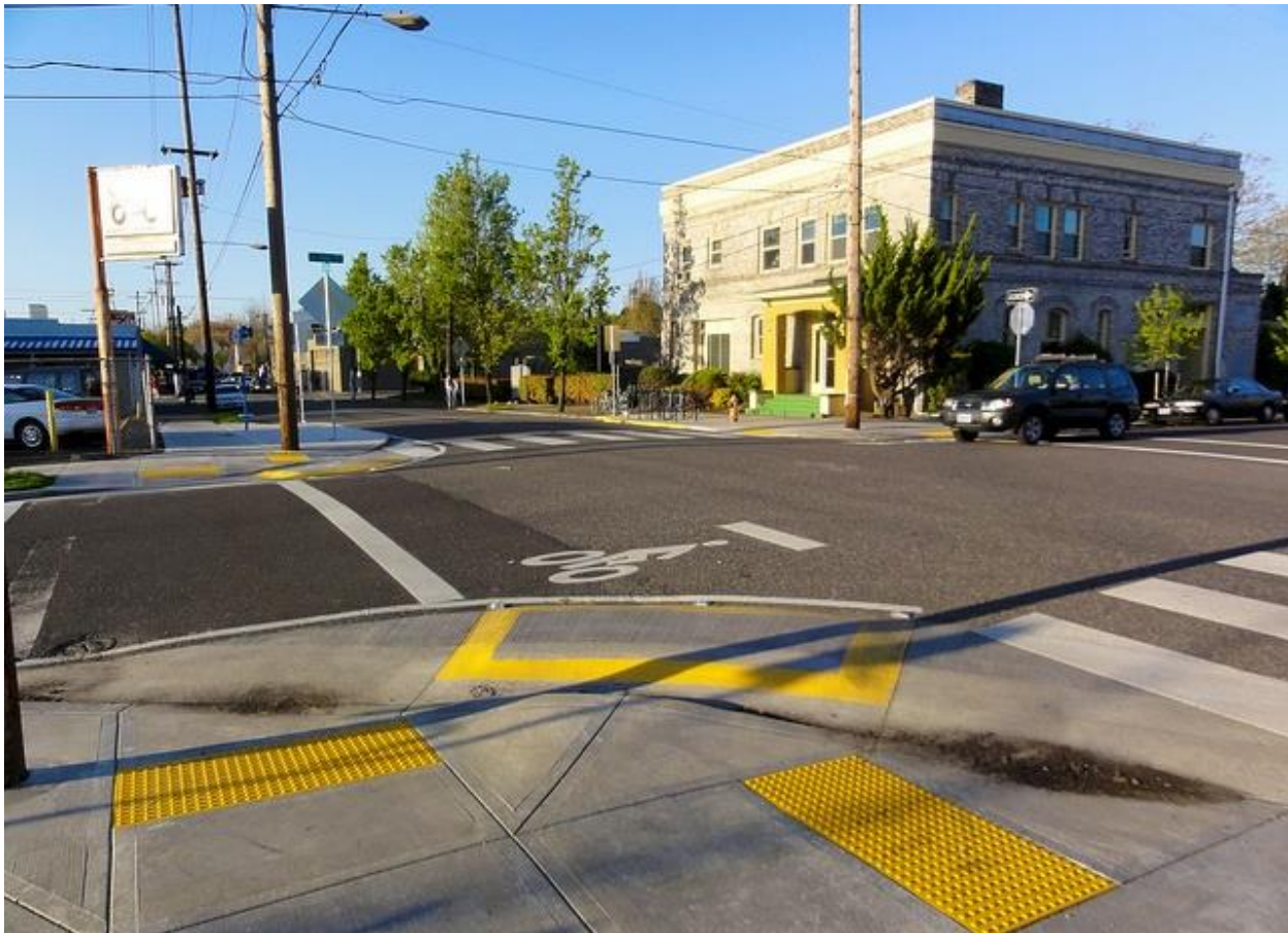
Figure 108: Mountable curb (Source: Google Images)
