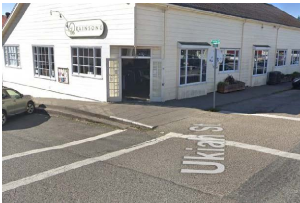
Figure 192: Southwest corner of Lansing Street and Ukiah Street intersection. (Source: Google Street View)
