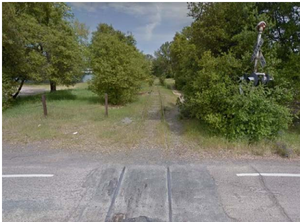
Figure 161: existing rail Line, looking north from Moore Street (Source: Google Street View)
