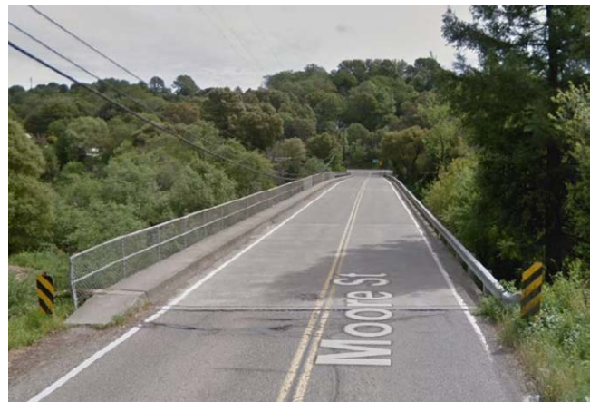
Figure 160: Moore Street Bridge with narrow shoulders and limited lighting (Source: Google Street View)
