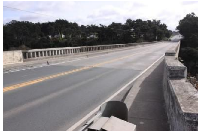
Figure 48: Hare Creel Bridge western sidewalk
