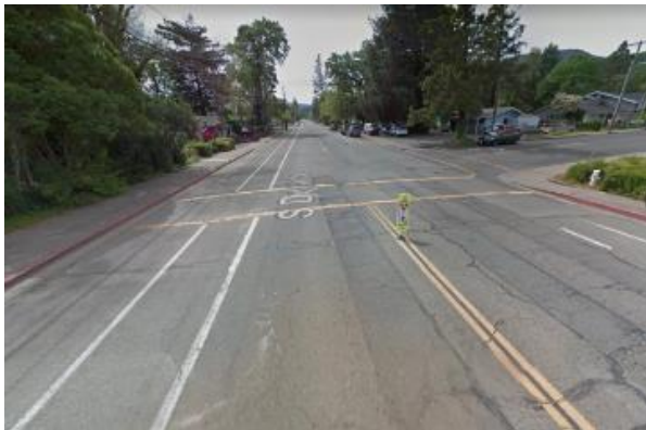
Figure 74: Intersection of Dora Avenue and Mendocino Avenue, Looking South (Source: Google Street View)
