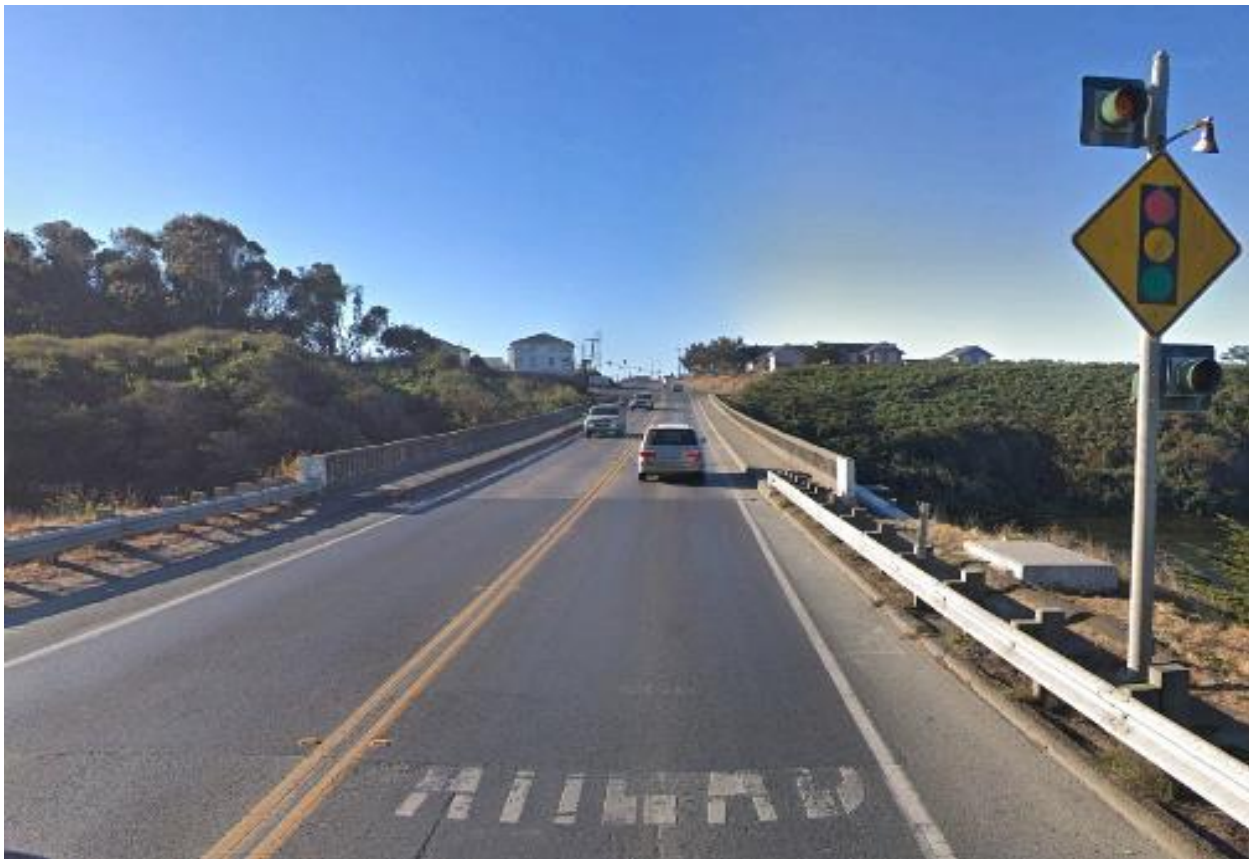
Figure 30: Highway 1 Pudding Creek Bridge, looking south (Source: Google Street View)
