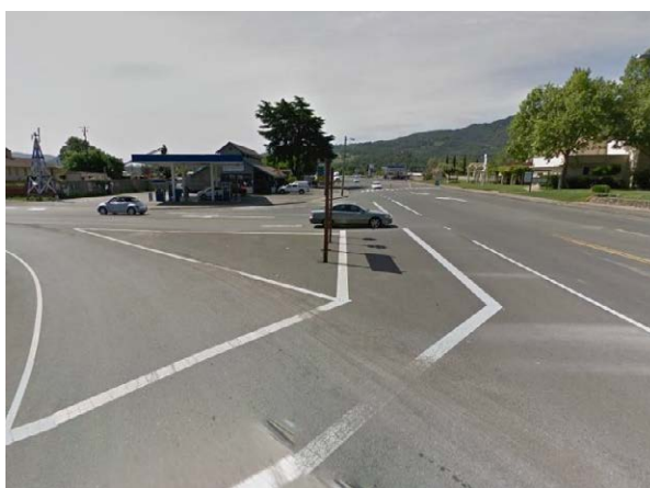
Figure 175: Intersection of Highway 101 and Highway 175, looking south (Source: Google Street View)
