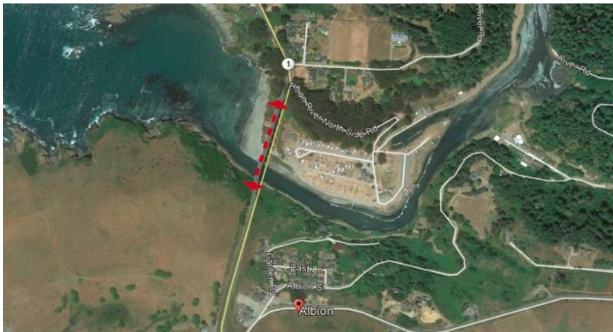
Map 69: Albion River Bridge (Source: Google Earth)
