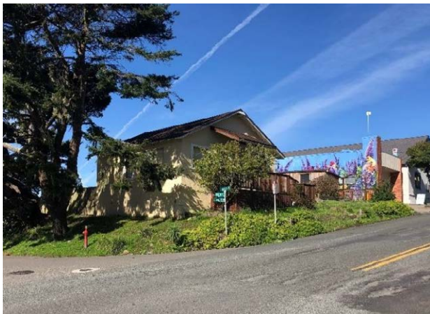
Figure 5: Corner of Iverson Ave. at Main St.
