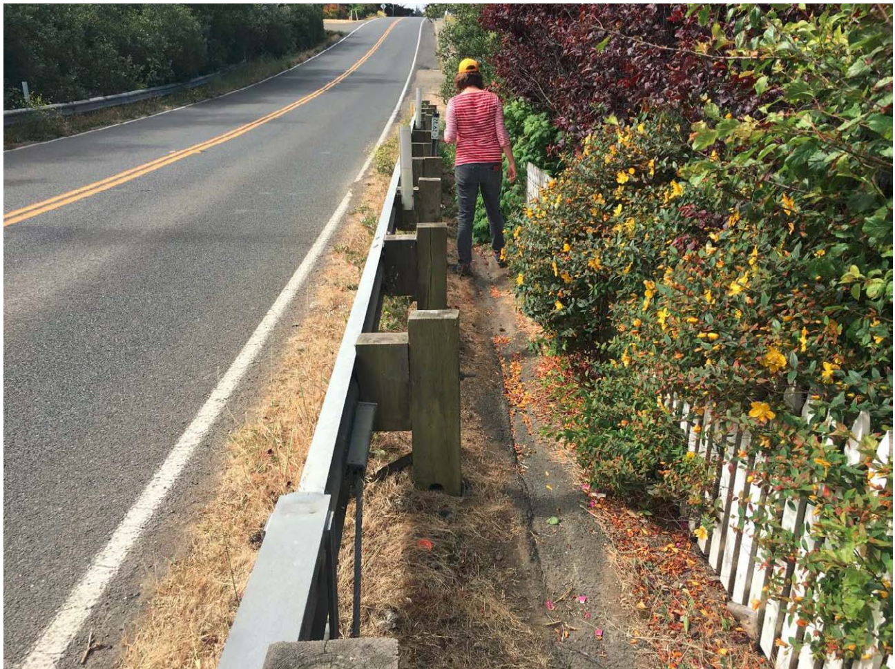
Figure 24: Pedestrian access gap on west side of Hwy 1 in Manchester
