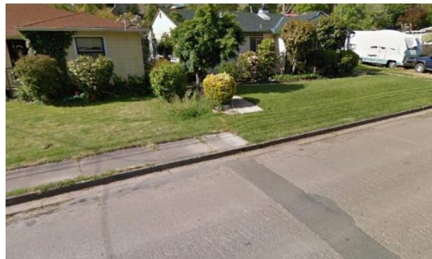
Figure 115: Section of West Mendocino Avenue without sidewalk (Source: Google Street View)
