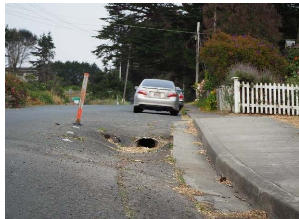
Figure 3: Open drainage along Riverside Drive
