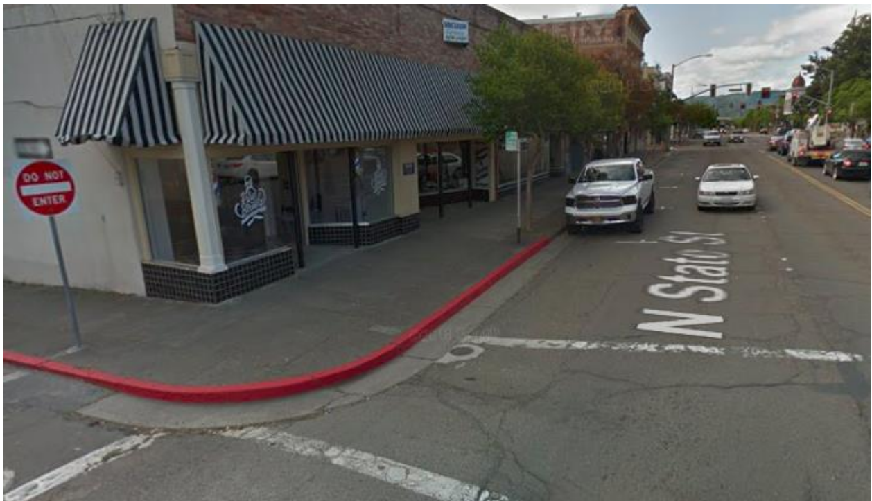
Figure 97: The intersection of North State Street and Smith Street lacks ADA accessible curb ramps (Source: Google Street View)
