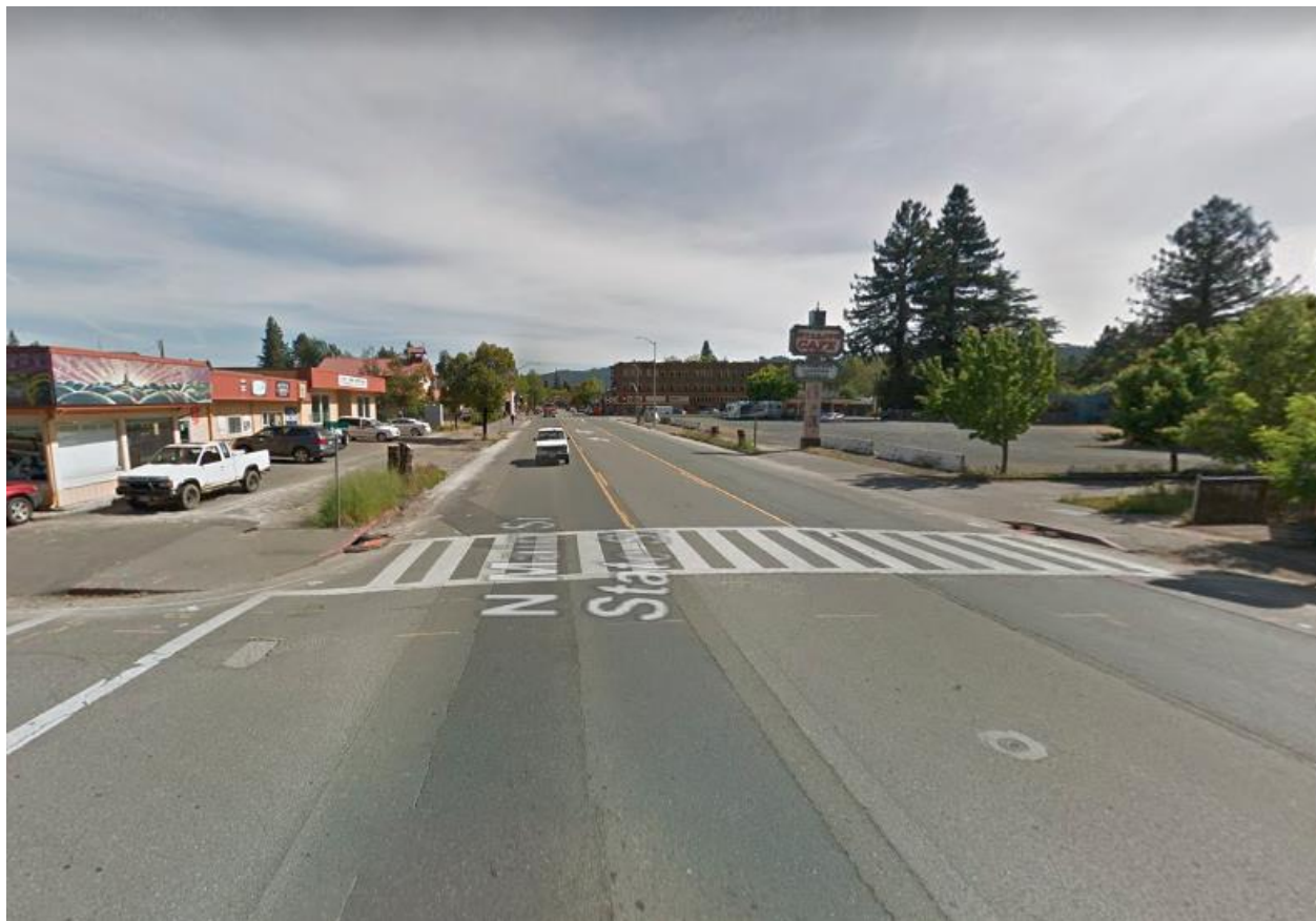
Figure 138: The intersection Redwood Highway with State Street has no lighting fixtures, look south (Source: Google Street View)
