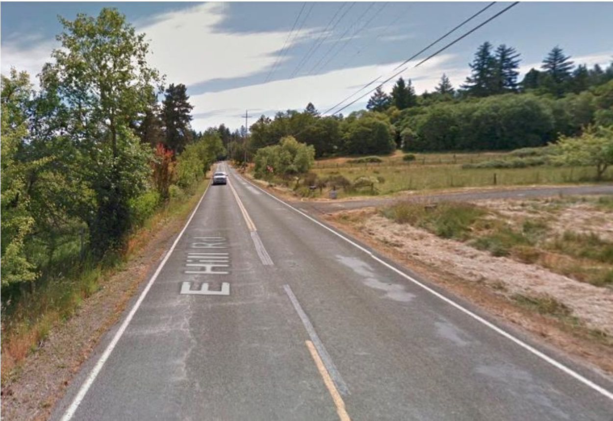
Figure 143: East Hill Road, near Highway 101 looking east (Source: Google Street View)
