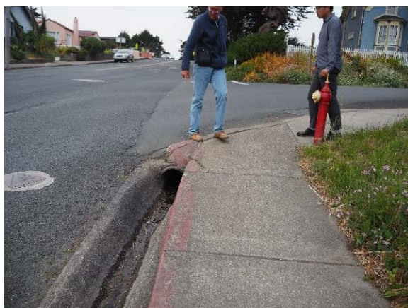
Figure 4: Open drainage along Main St./Hwy 1
