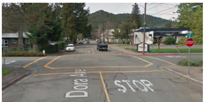
Figure 60: Intersection of Dora Avenue and Willow Avenue, Looking North (Source: Google Street View)
