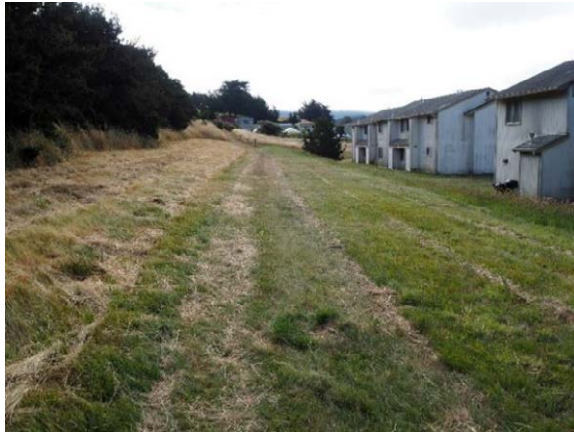
Figure 14: Trail behind Point Arena Village Apartments
