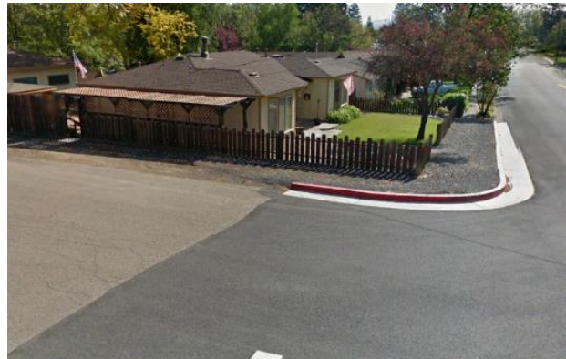
Figure 117: Intersection of Easy Street and Redwood Avenue is missing sidewalk and curb ramps (Source: Google Street View)
