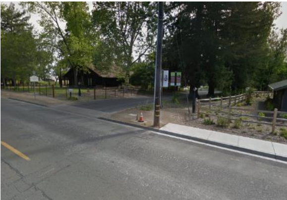
Figure 68: Main Street, between Clay and Cleveland Street with sidewalk missing (Source: Google Street View)
