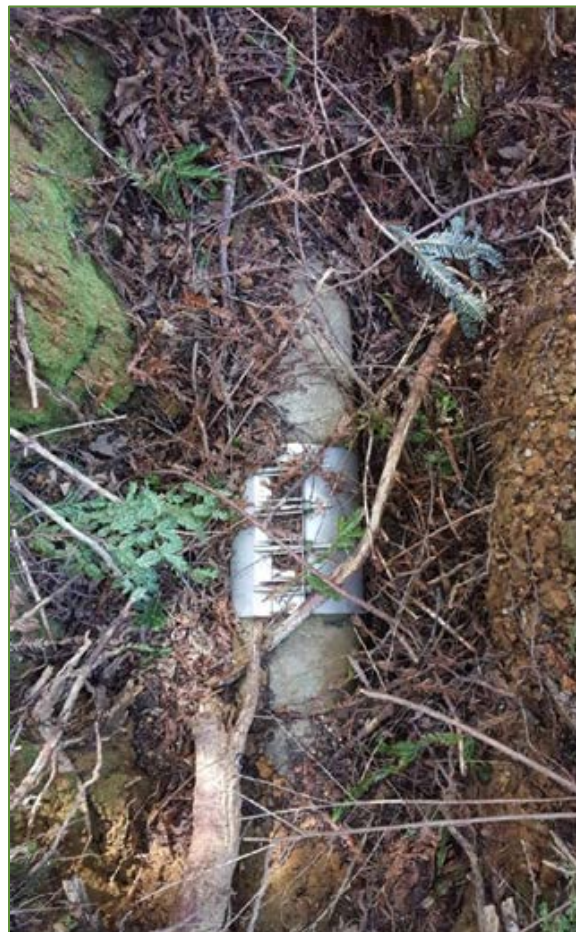
Clamp Repair of Exposed Pipe
