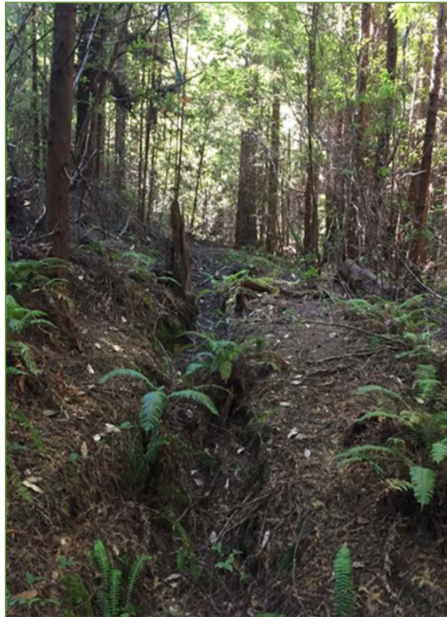
Existing Sunken Pipe Trench
