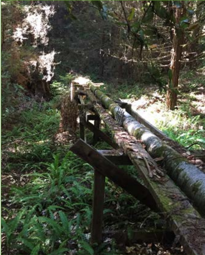
Phase V Trestle
