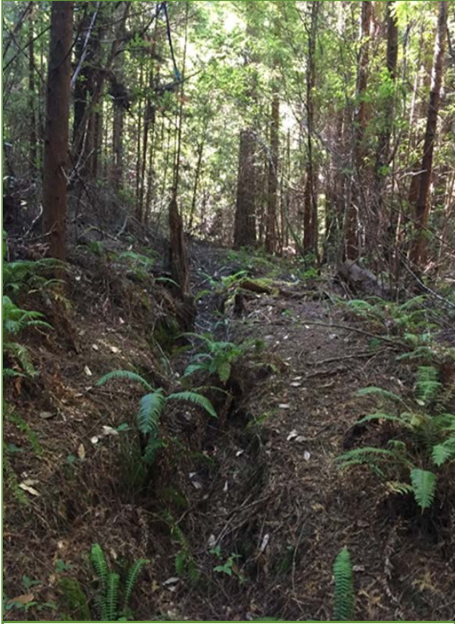
Existing Sunken Pipe Trench
