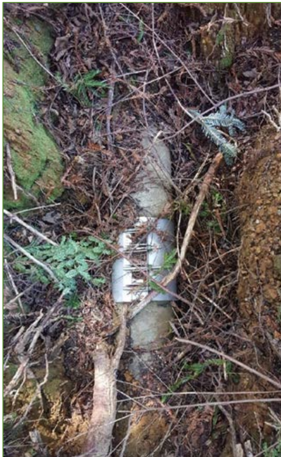
Clamp Repair of Exposed Pipe
