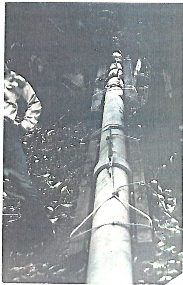
P-23 10" PIPELINE - ALIGNMENT UP NORTH BANK OF COVINGTON GULCH →
