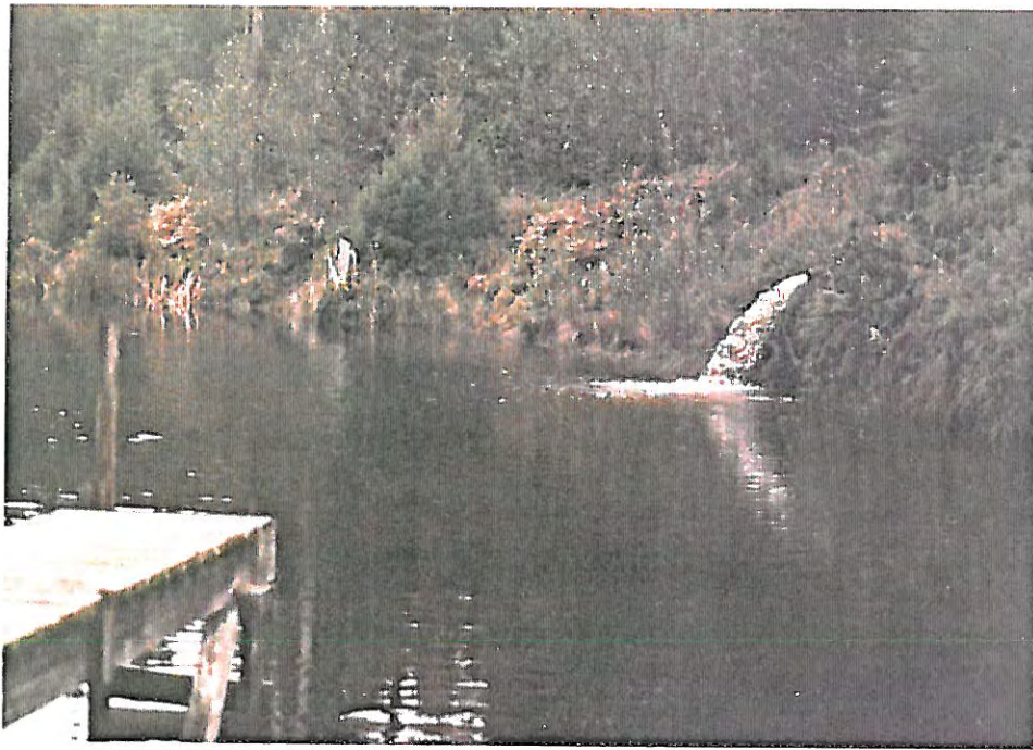
▲ P-24 SIMPSON PIPELINE 6" DISCHARGE INTO NEWMAN RESERVOIR - JANUARY 1985
