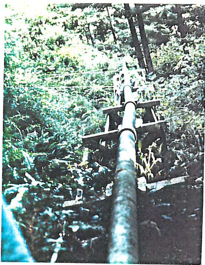
◀ P-9 TRESTLE # 8 LOOKING NORTH
