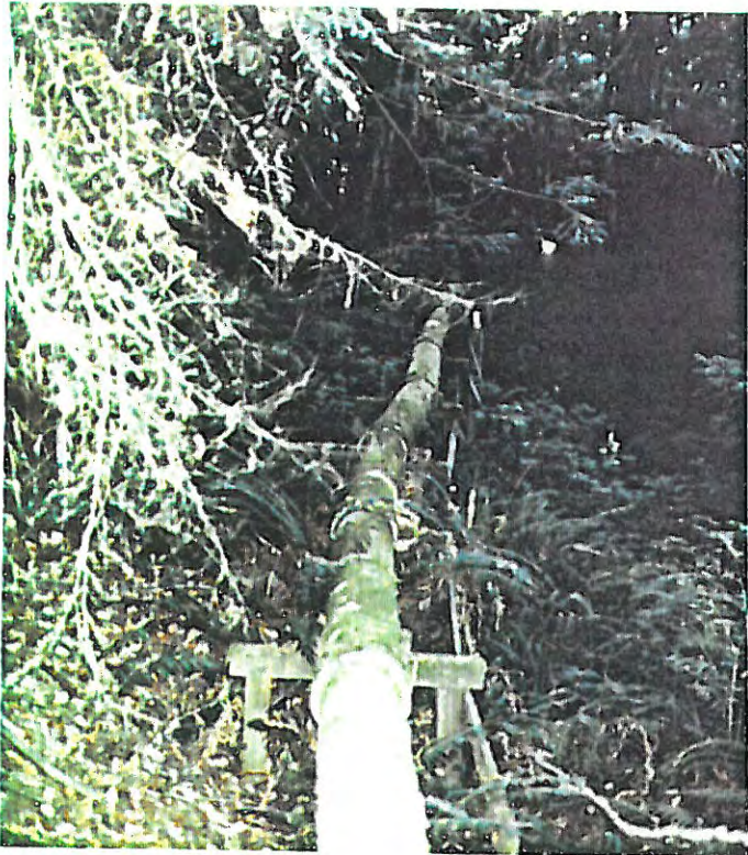
◀ P-7 TRESTLE #1 - DOWNSTREAM OF SIMPSON PIPELINE
