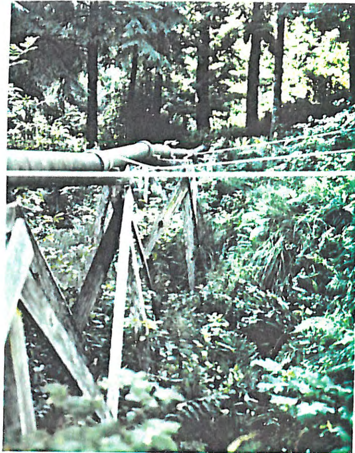
P-10 TRESTLE # 8 ▶ LOOKING SOUTH
